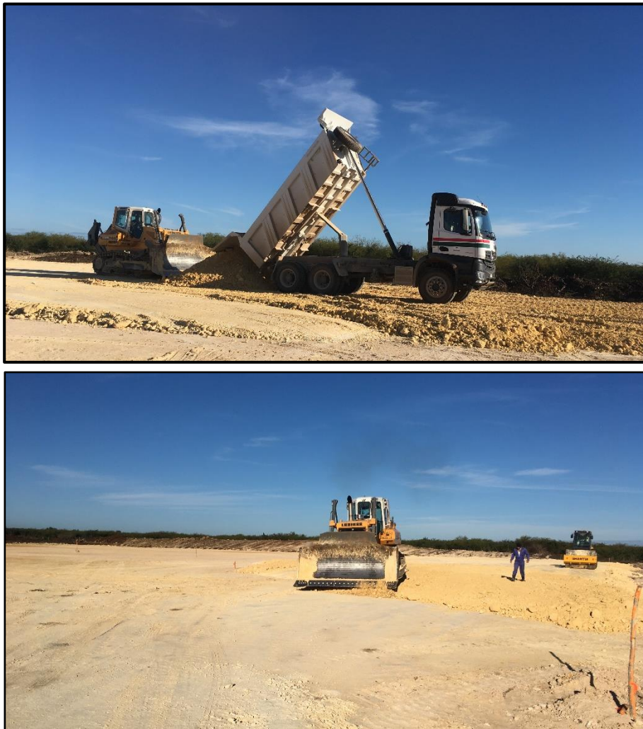
Figure 1 – Civil works are more than half complete for Alameda-1
