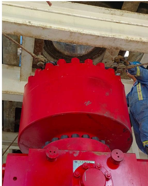
*Figure 2 - BOP installed and tested*
