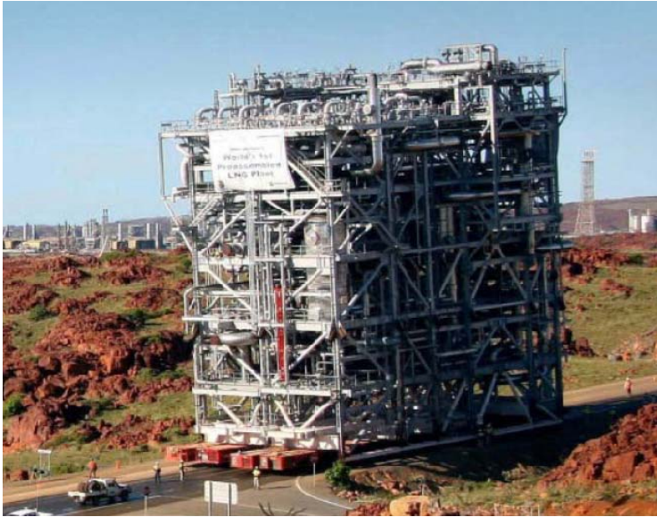
A NWS Train 5 (4.4 Mtpa) module. Pluto I (4.3 Mtpa) has 264 modules .
