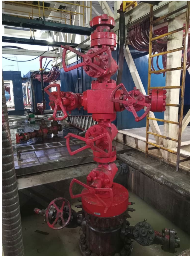
Figure 2 - Alameda-2 completion successfully run
