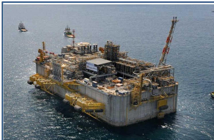
ExxonMobil Adriatic Re-gas terminal
