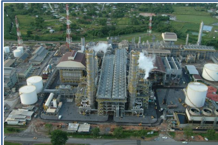
DPT M5000 plant - Trinidad
