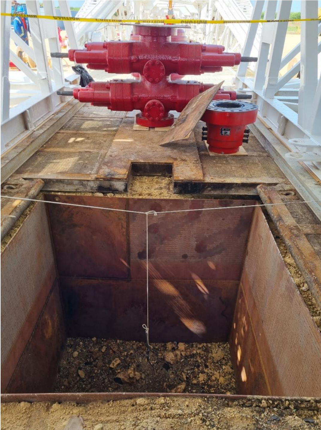
Figure 2 – Preparation of the BOP stack prior to installation
