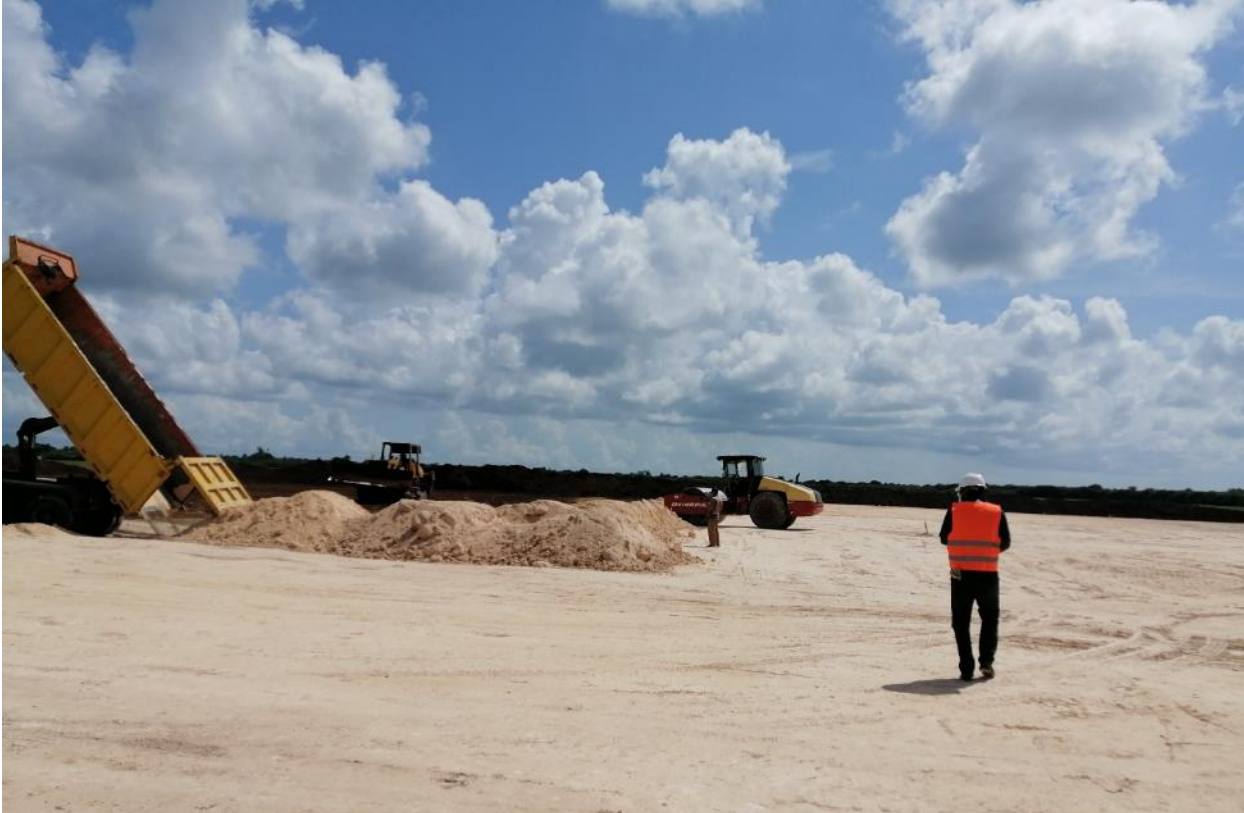
Figure 3 – Build-up of the Zapato-1 well pad continues
