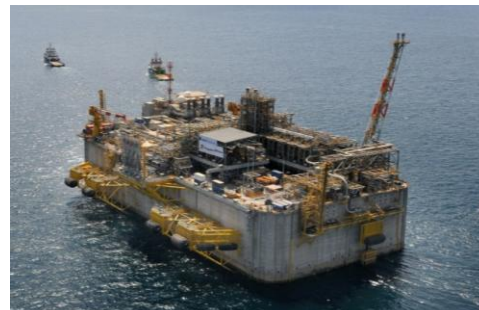
ExxonMobil's Adriatic Re-gas terminal on CGS. Barge becomes island and storage
