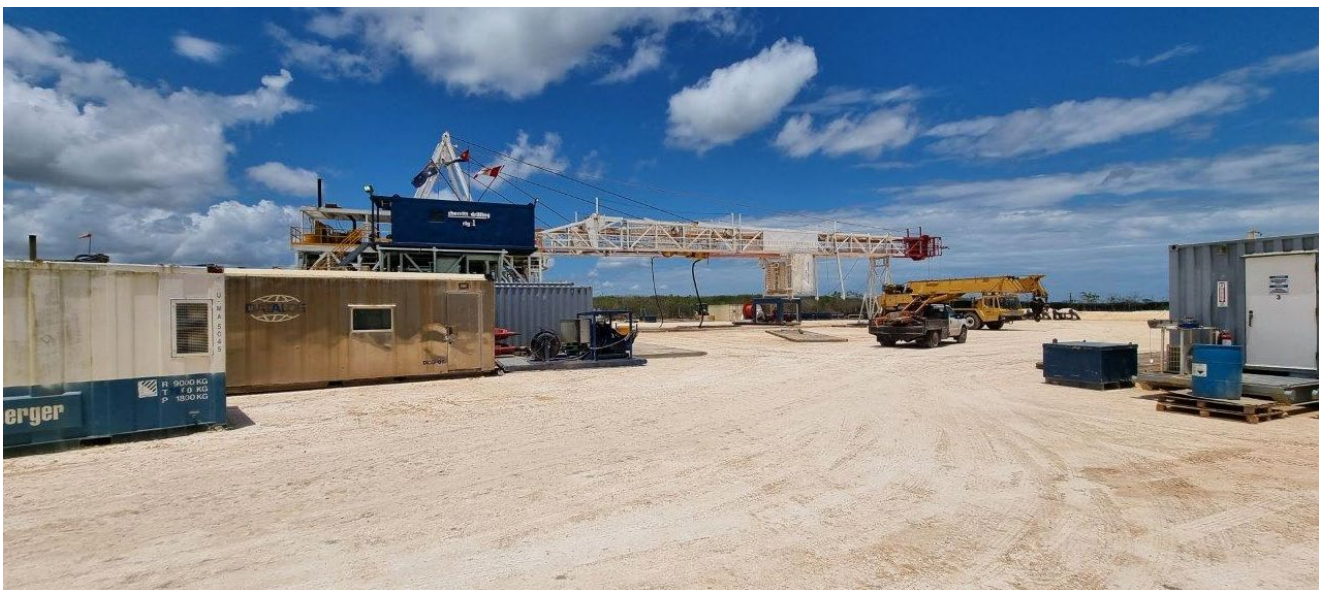
Image 1: Rig installation works underway at Zapato-1 drill site
