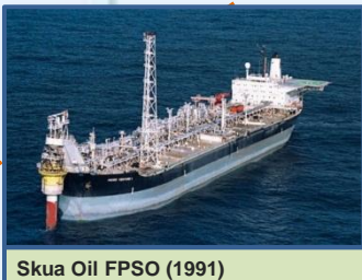
Skua Oil FPSO (1991)
