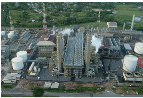
Process plant based on Davy Process Technology plants operating in Trinidad
