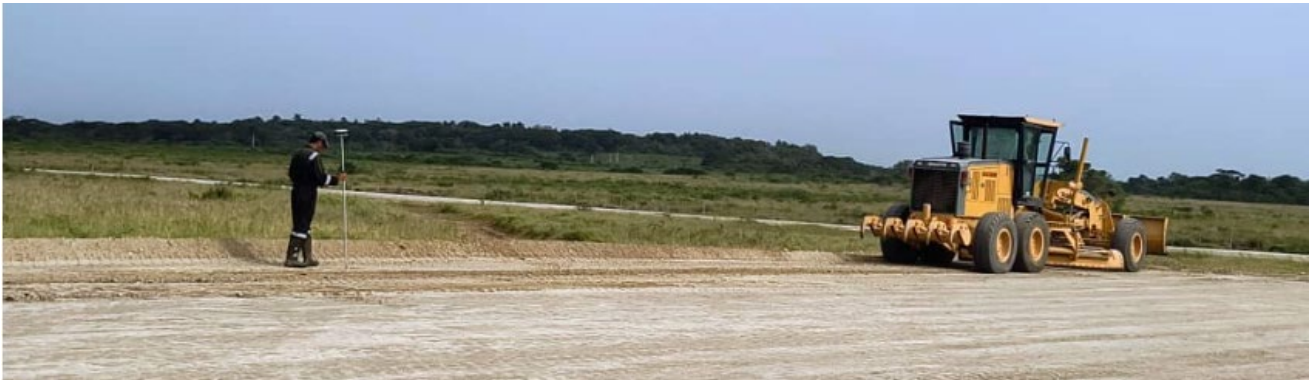
Figure 2 – Construction of pad for Amistad-3 nearing completion during the reporting period.
