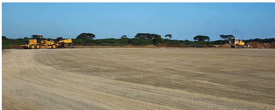
Figure 3 - Construction of pad for Amistad-3 was completed.
