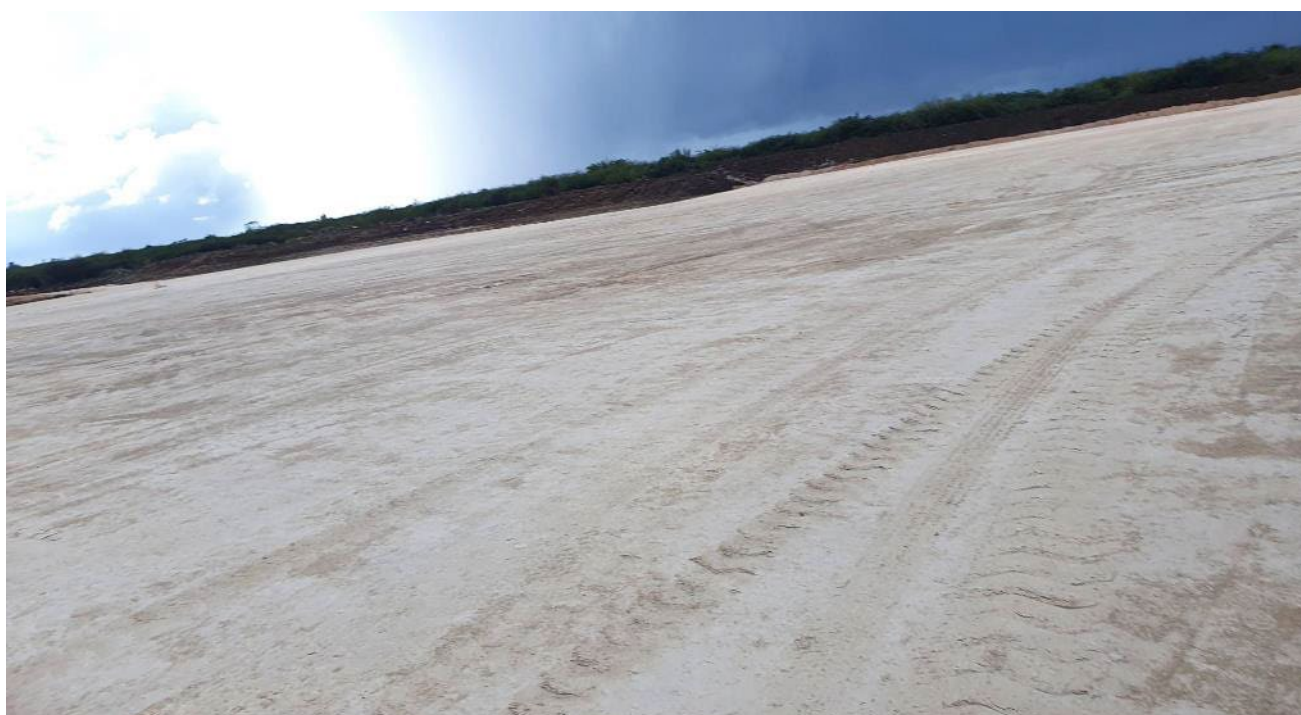
Figure 1 - Alameda pad ready for drilling operations
