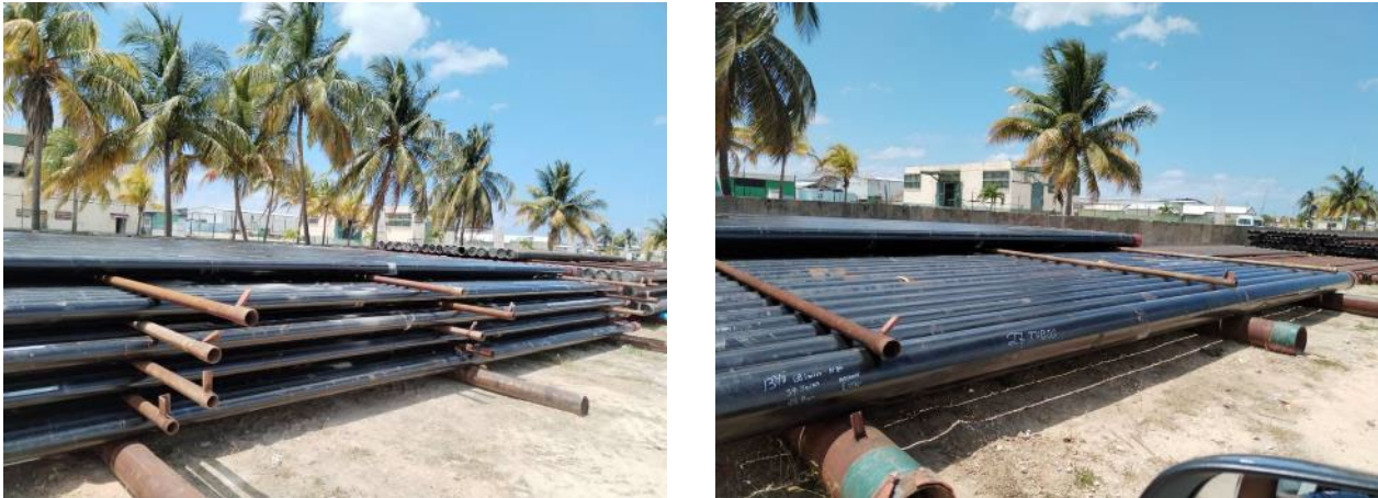
Figure 2 – Casing racks in Melbana’s laydown yard in Varadero, Cuba
