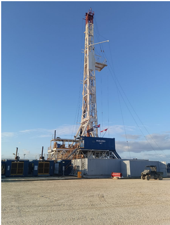
Drilling ready to start.
