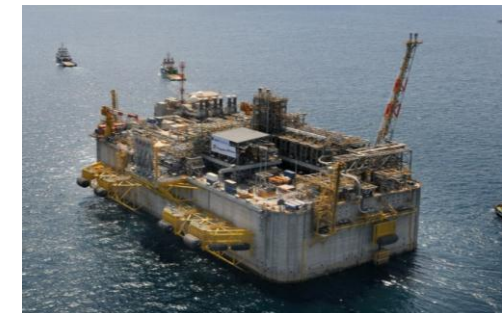
CGS has same footprint as ExxonMobil's Adriatic Re-gas terminal CGS
