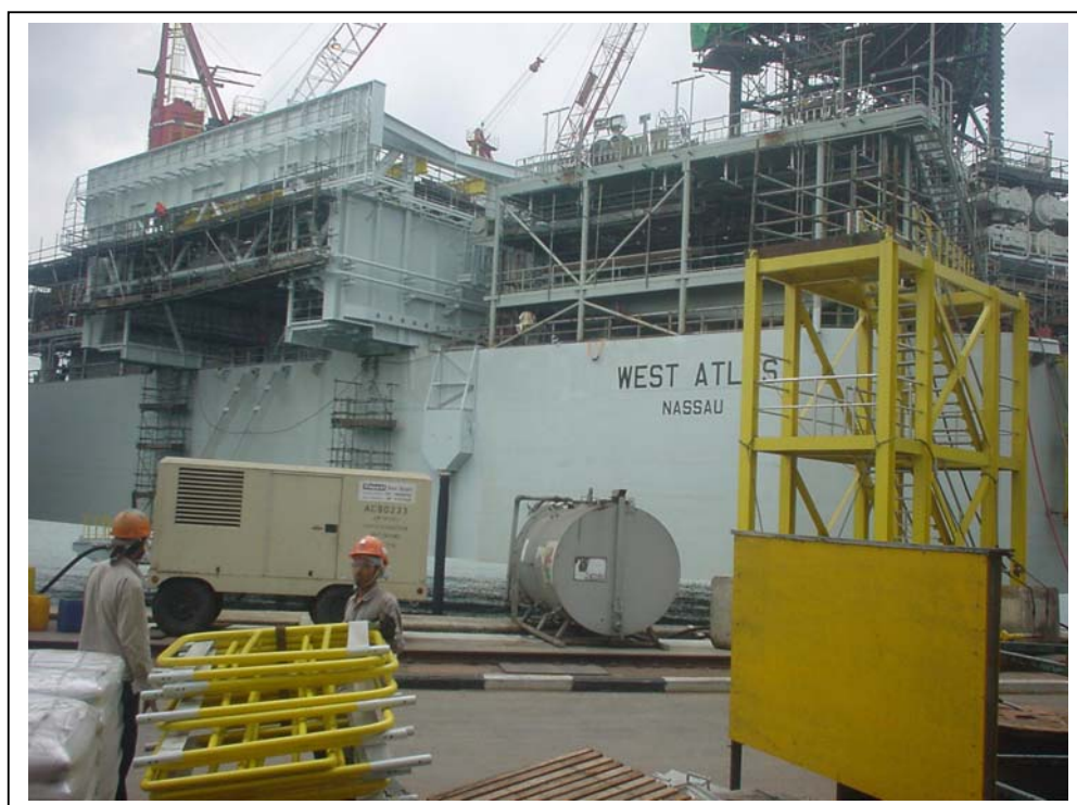
West Atlas jack-up rig construction in fit-out stage
