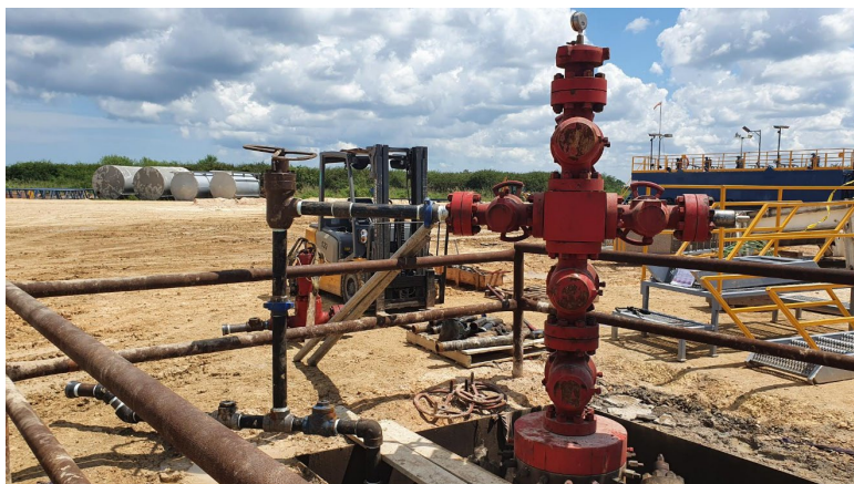
Figure 5– Establishment of equipment for early production from Alameda-2 Unit 1B
