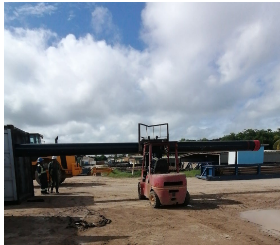
Figure 4– Additional casing load-in
