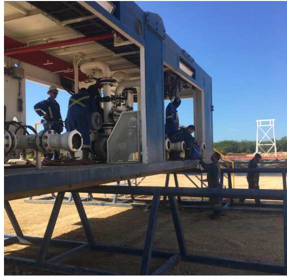
Figure 2 – Rig set up for Alameda-3
