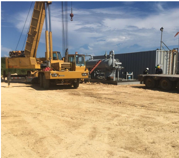
Figure 3 – Separator move for Alameda-3
