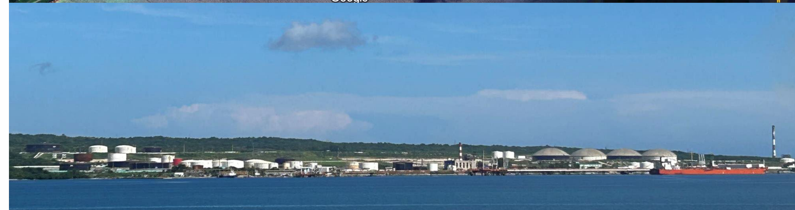
Matanzas Port and Refinery facilities as seen from the bay
