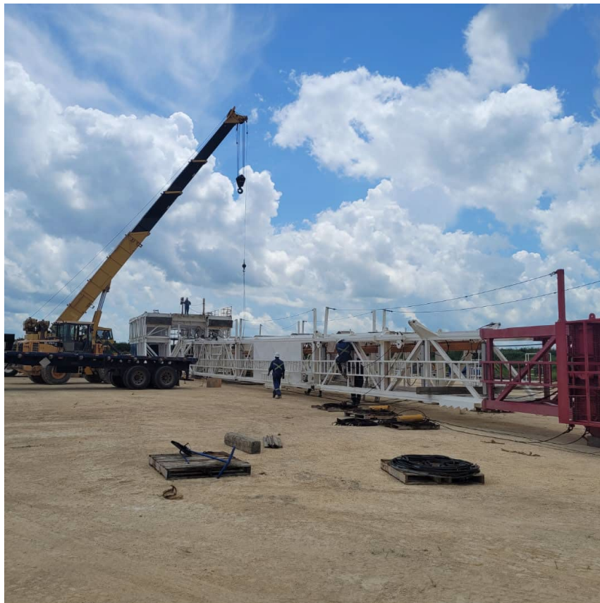
Figure 1 – Delivery of components of drilling rig
