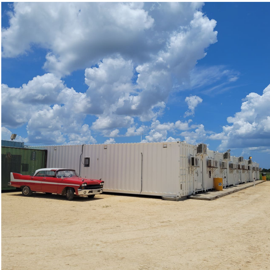
Figure 3 – Camp now installed and operational
