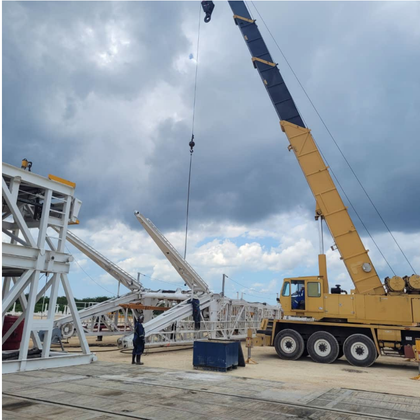
Figure 2 – Preparing for installation of drilling rig
