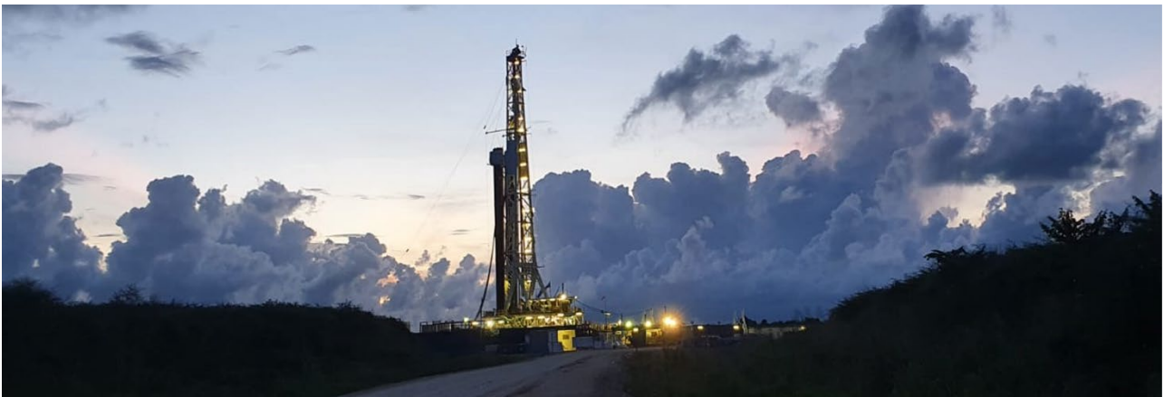
Figure 1 - Rig at dusk at the Alameda-1 site
