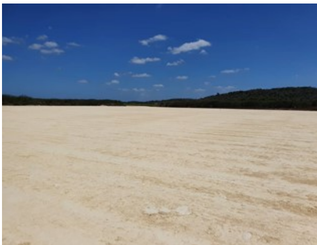
Figure 1 - Completed well pad at Alameda-1
