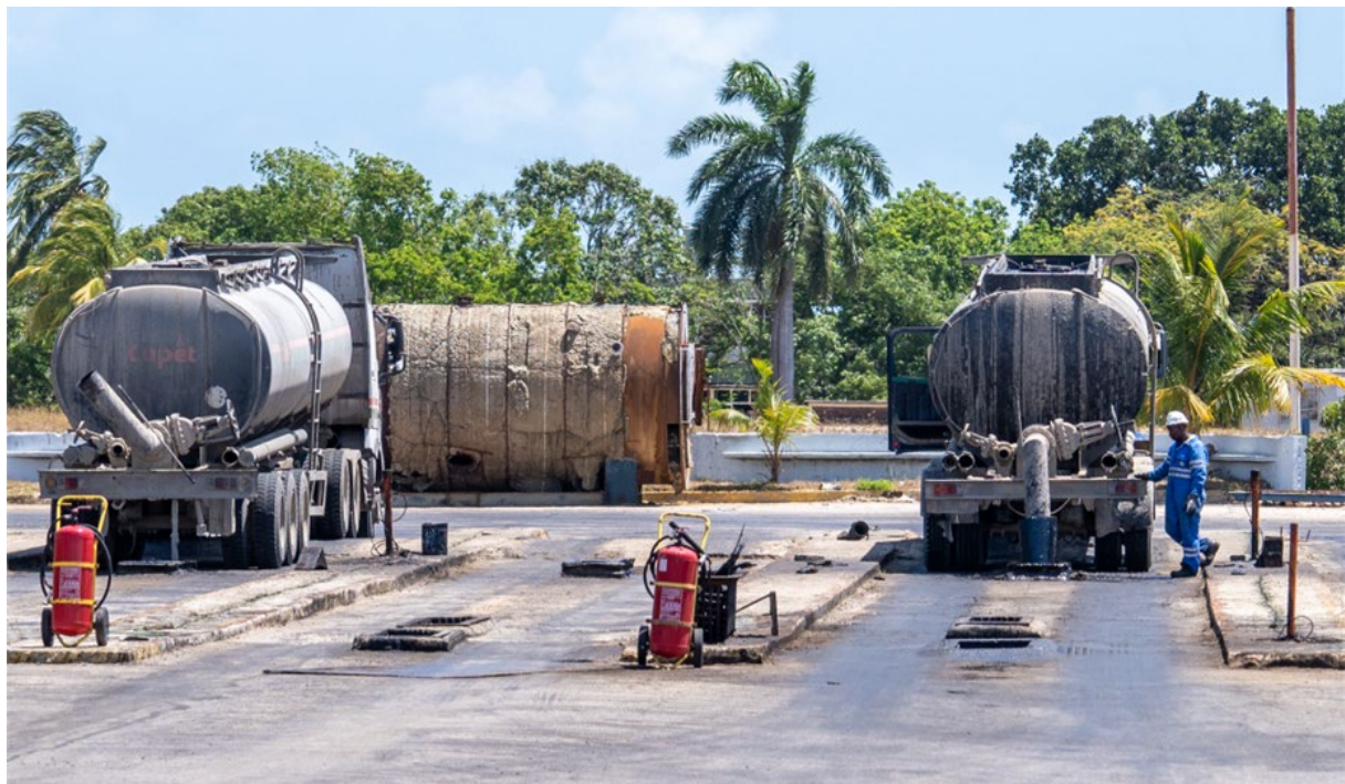
Figure 8 - Oil unloading at Varadero Tank Battery
