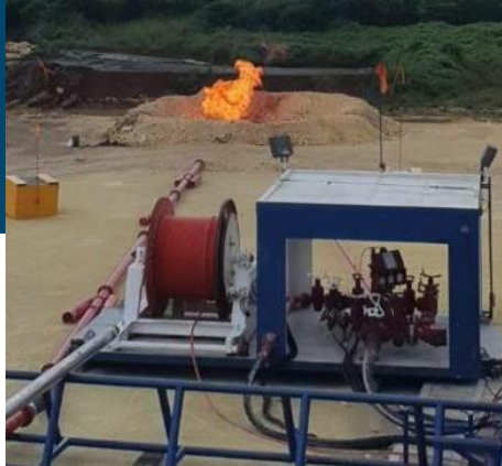
Flaring whilst drilling Alameda-1 (2022)
