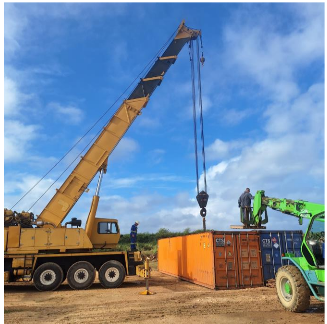
Delivery of workover chemicals
