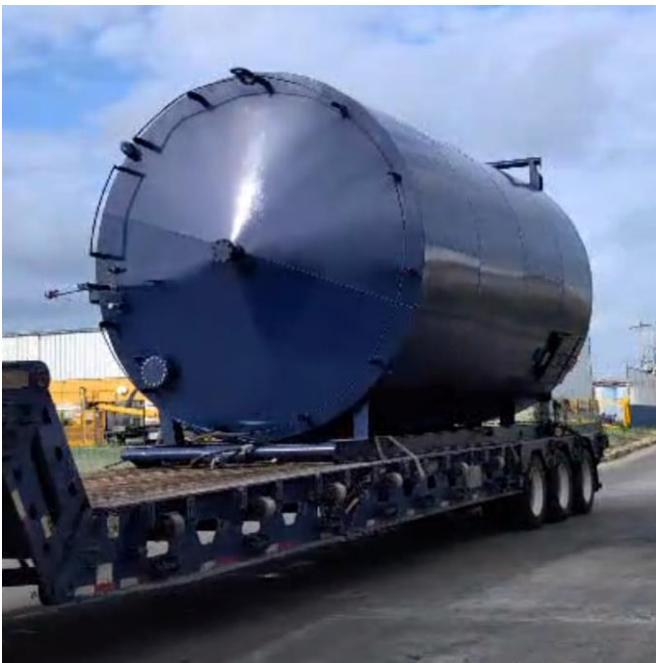
Storage tanks being delivered to site
