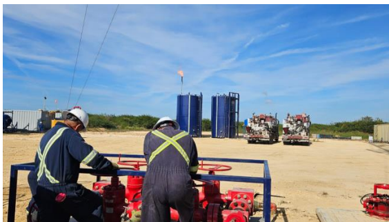
Inspecting equipment integrity
