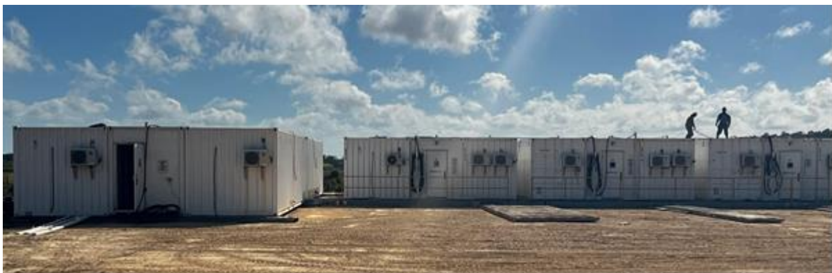
Figure 3 - Camp construction near completion
