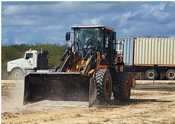
Figure 1 - Surface preparations complete
